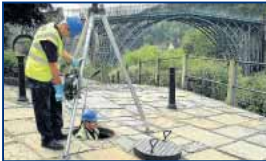
The Fabweld Steel Products team at work in Ironbridge
